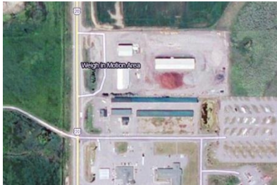
Project Site (Pre-Construction)
